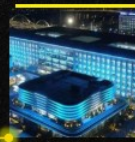
Lotus Technology Research Institute Ningbo, China Electric architecture, charging & power system
