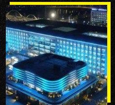
Lotus Technology Research Institute Ningbo, China Electric architecture, charging & power system
