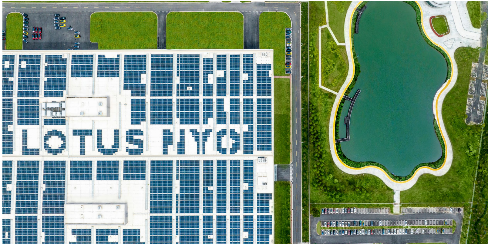
Photovoltaic power stations in Lotus Global Smart Factory
